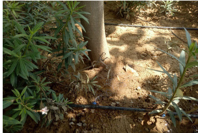
Storm water drain and Drip Irrigation
